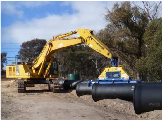
**Figure 1 Pipe being strung along the corridor for installation**
